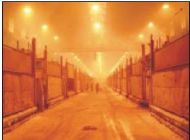
HSS Pot Line at Hiralud Smelter, Hindalco
