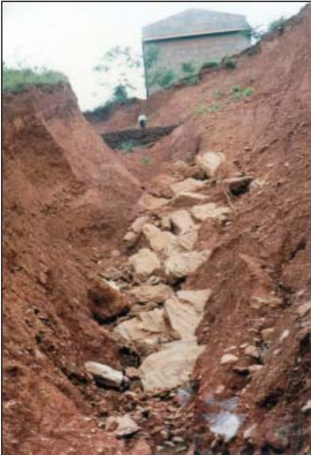
Bund to Arrest Soil Erosion, NALCO
